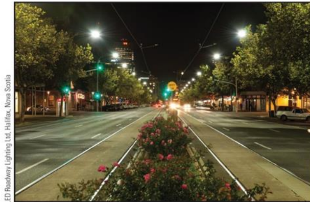
Figure 17.6: Conversion of streetlights on King William Street, Adelaide, Australia from (top) high-pressure sodium fixtures to (bottom) LED streetlights.
